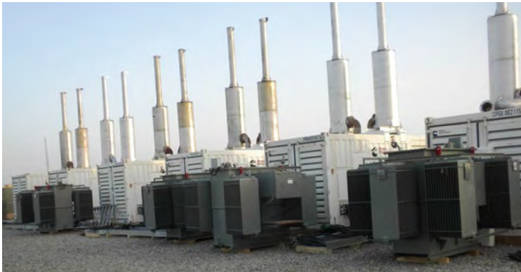
MOBILE PACKAGE SUBSTATION 33 kV / FEWA
